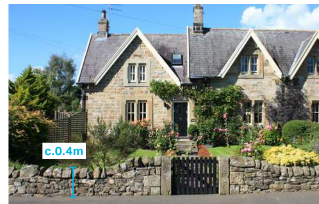
Figure 78: Positive example of low stone wall boundaries, tying in to natural stone gate posts and wooden gate.
