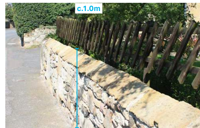
Figure 76: Taller boundaries can be used where there is a need for privacy e.g. back garden facing on to road or side boundaries, although lower walls are often most suitable for street facing façades.
