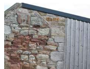
metal roof on outbuilding
