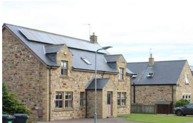
Figure 90: Example of retrofitted solar panels in Longhoughton.
