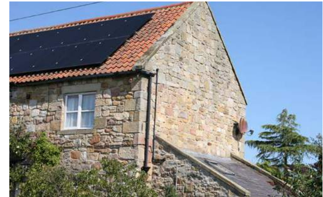
Figure 91: Example of retrofitted solar panels in Longhoughton.
