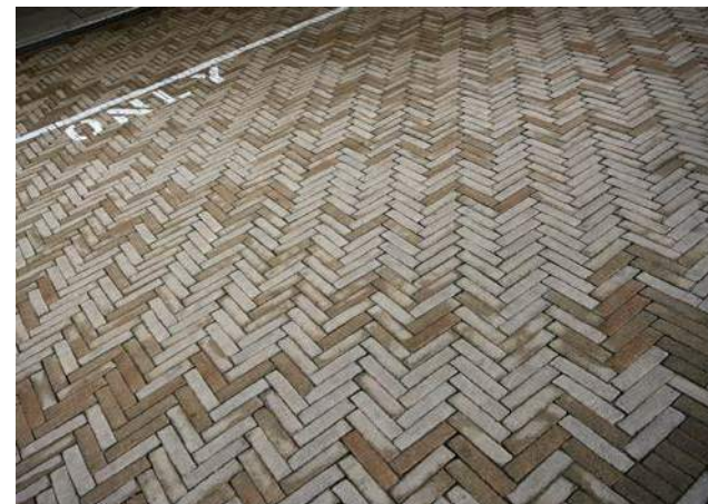
Figure 94: Permeable Paving (Hardscape)
