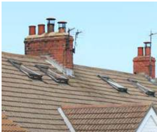
Brick clay pot chimneys
