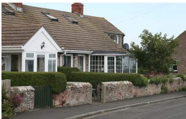
Figure 77: Positive example of low stone wall boundaries, with additional interest provided by the addition of vegetated boundaries, either dividing properties or adding privacy where facing onto a road.
