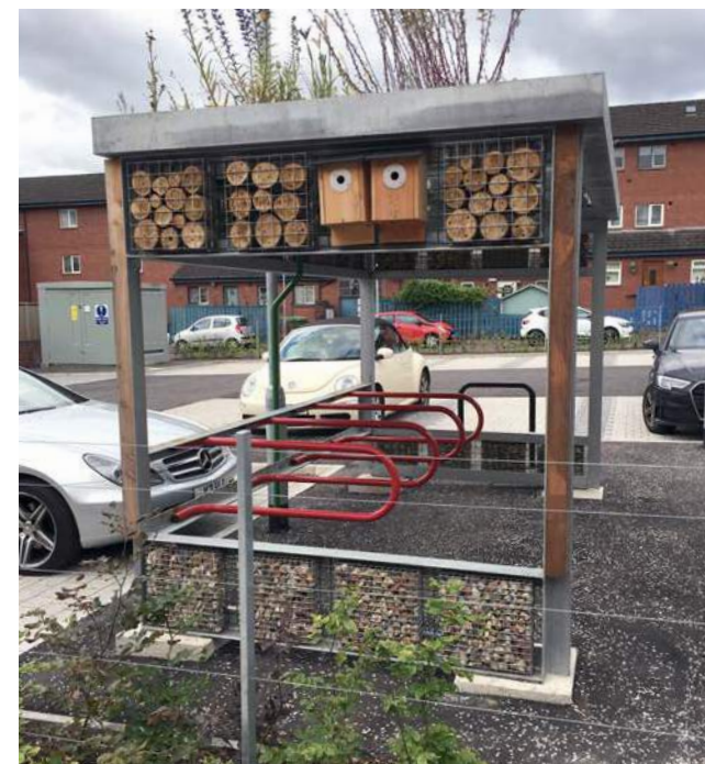
Figure 83: Bike shelter with habitat provision and green roof, serving commercial and multi-occupancy flat development, Glasgow.
