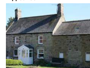
Typical pitched roof
