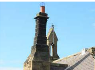
Natural stone chimneys
