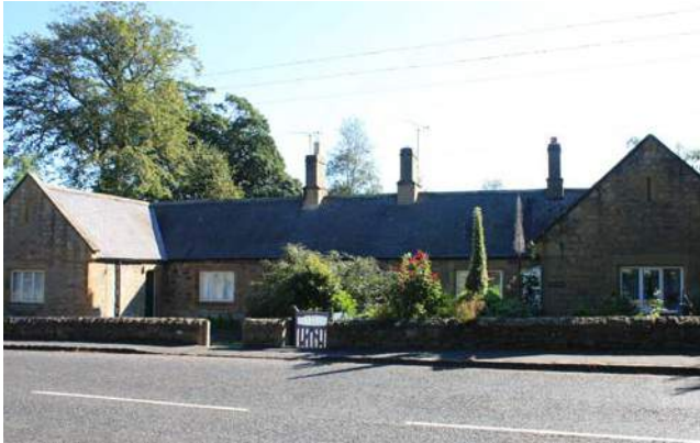
Figure 4: Longhoughton: Example of paired bungalows
