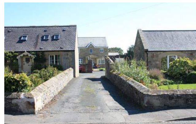
Figure 66: Opportunities for back-of-plot development can contribute to raising density and enhancing visual interest.
