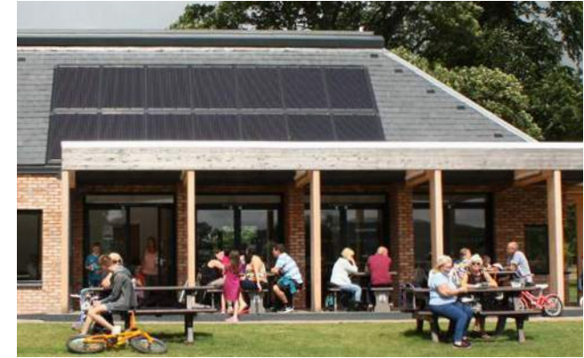
Figure 89: Solar Panels on a new build at Levensgrove Park, Dumfries.
