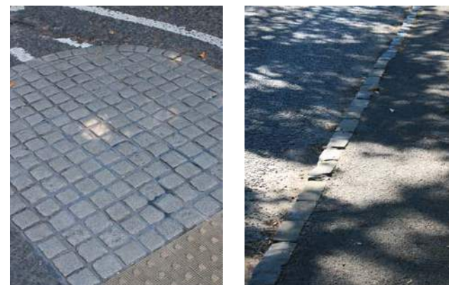
Figure 47: The use of natural stone materials, such as these square setts, and natural stone kerbs, adds quality where it appears and should be used in new development.
