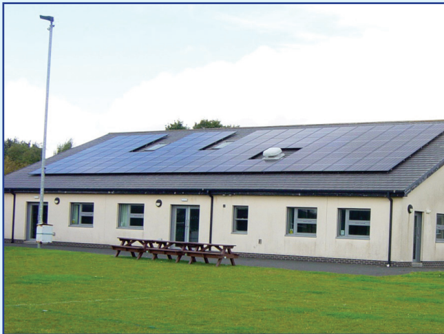
76 solar panels have been fitted to the roof at Westfield Park in a move towards energy self-sufficiency
